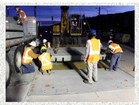
This was the second Super Slab project in Utah, and consisted of repairs to I-15 NB and SB, the major transportation corridor north of Salt Lake City between the Wasatch range on the east and the Great Salt Lake to the west. Precasting was completed by a local fabricator, Mountain West Precast, of Ogden. All repair slabs were 6' long. Due to the presence of many areas requiring multiple slabs, the contractor was able to install as many as 20 slabs per night.
